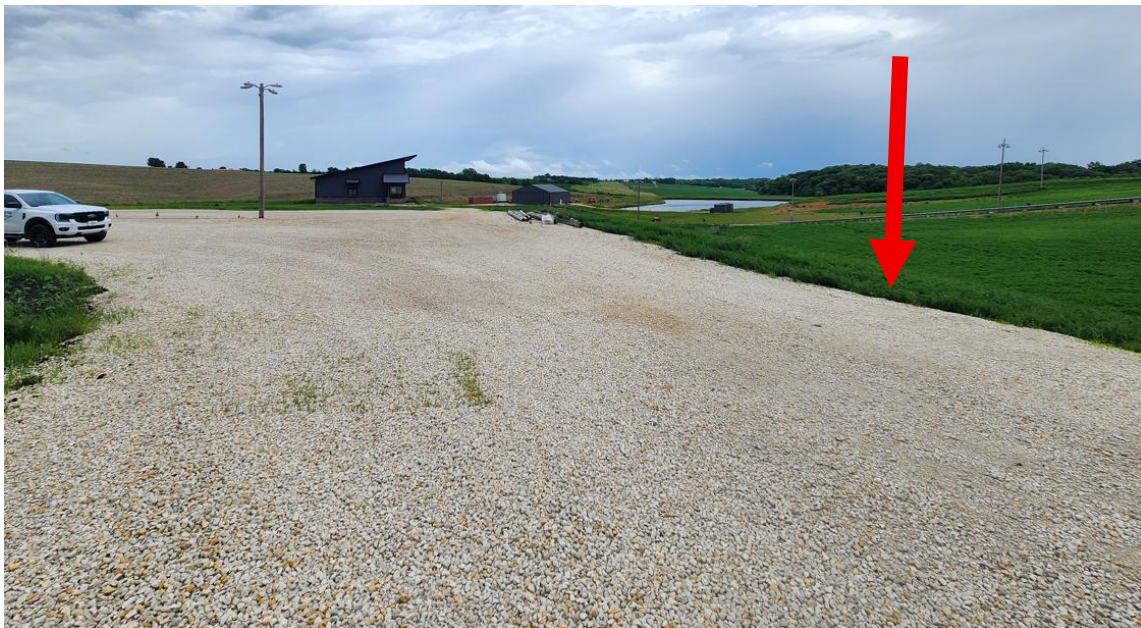
The South edge of the parking lot, where approximately 0.8' to 7.8' of fill was designed
