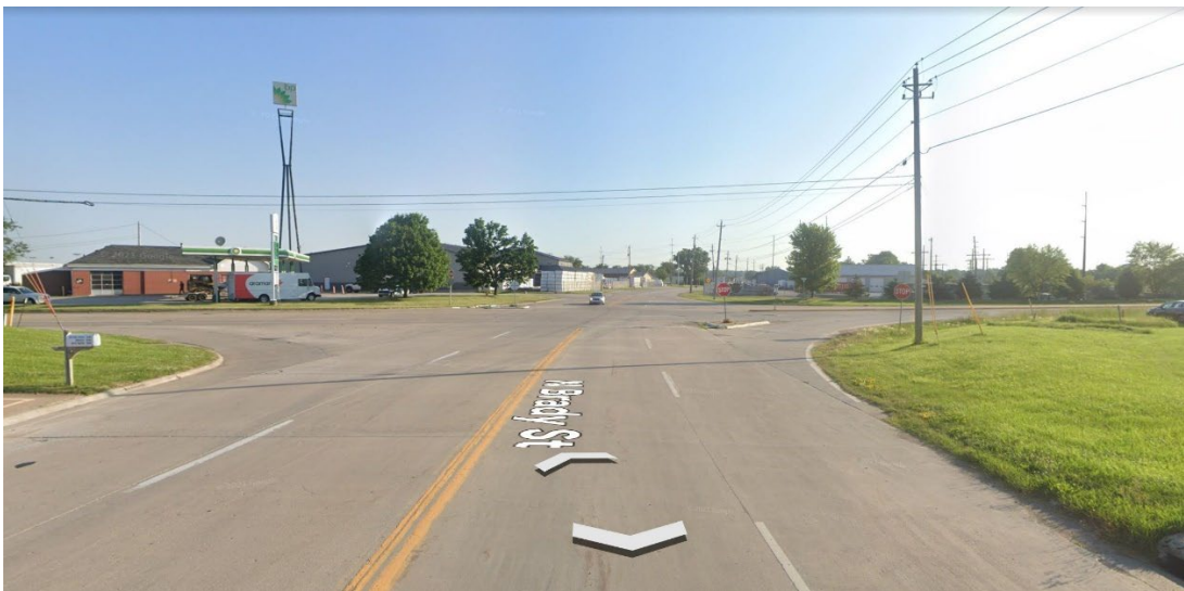
Figure 12 –Roadway Characteristics –South leg of the 210 th Street and Brady Street Intersection Looking North
