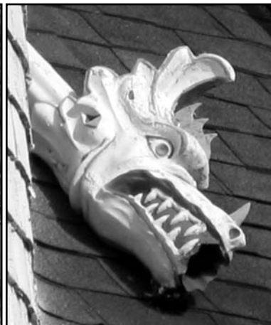
RIGHT: Gargoyle gutter on the roof
