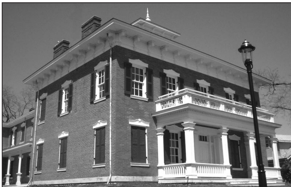
Current photo of the Antoine LeClaire House. Renovations coming right along!
