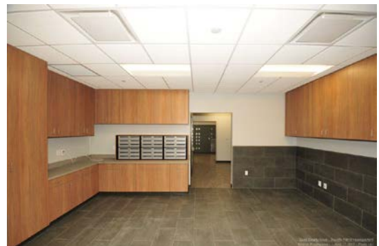
Patrol Remodel (Lobby)
