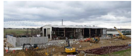
Scott County Waste Commission Single Stream remodel
